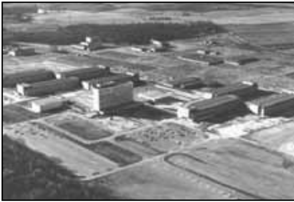
This overview, shot in 1966, of NBS's magnificent new campus at Gaithersburg, MD, has served as home for NBS/NIST since their move from downtown. It was designed to house superior facilities for industry conferences across the many constituent groups that NIST serves.
