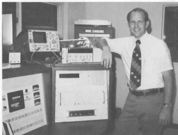
Tom Nebel of the HP St. Louis office prepares to fire up the atomic clock, using a frequency counter and an HF receiver to synchronize it with the NBS atomic clock in Boulder, Colorado.
