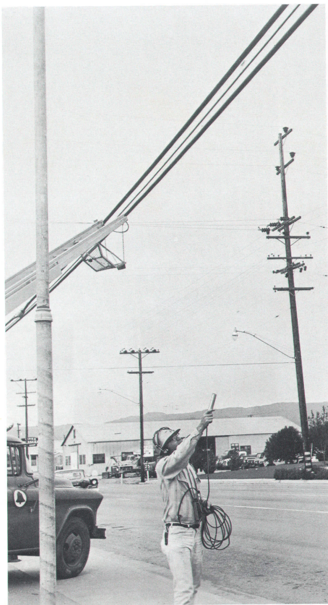
Ultrasonic detection of leaks in pressurized telephone cables has eliminated old-fashioned soap-bubble method. Leaks can usually be heard from the ground, often from a truck driving along the cable path. Translator responds only to sounds between 36 kHz and 44 kHz and is not affected by audible traffic noises.
